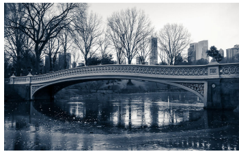
2 Bow Bridge over the...
